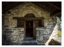
This Lombard Romanesque church was consecrated on 23 January 1164, according to the deed of consecration found inside the altar. Built on a rectangular plan and with a semicircular apse, it has a belfry with two openings which takes up the whole width of the west wall. The main door, in the west wall and decorated with a toothed frieze, is protected by a porch from a later time, from which one can see a magnificent panorama
